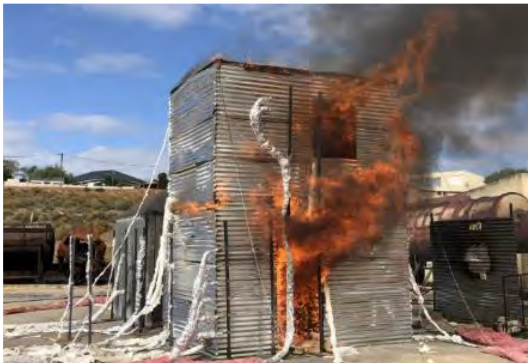
Figure 6-13: Full-scale fire test on a double storey dwelling showing the intensity of the fire
