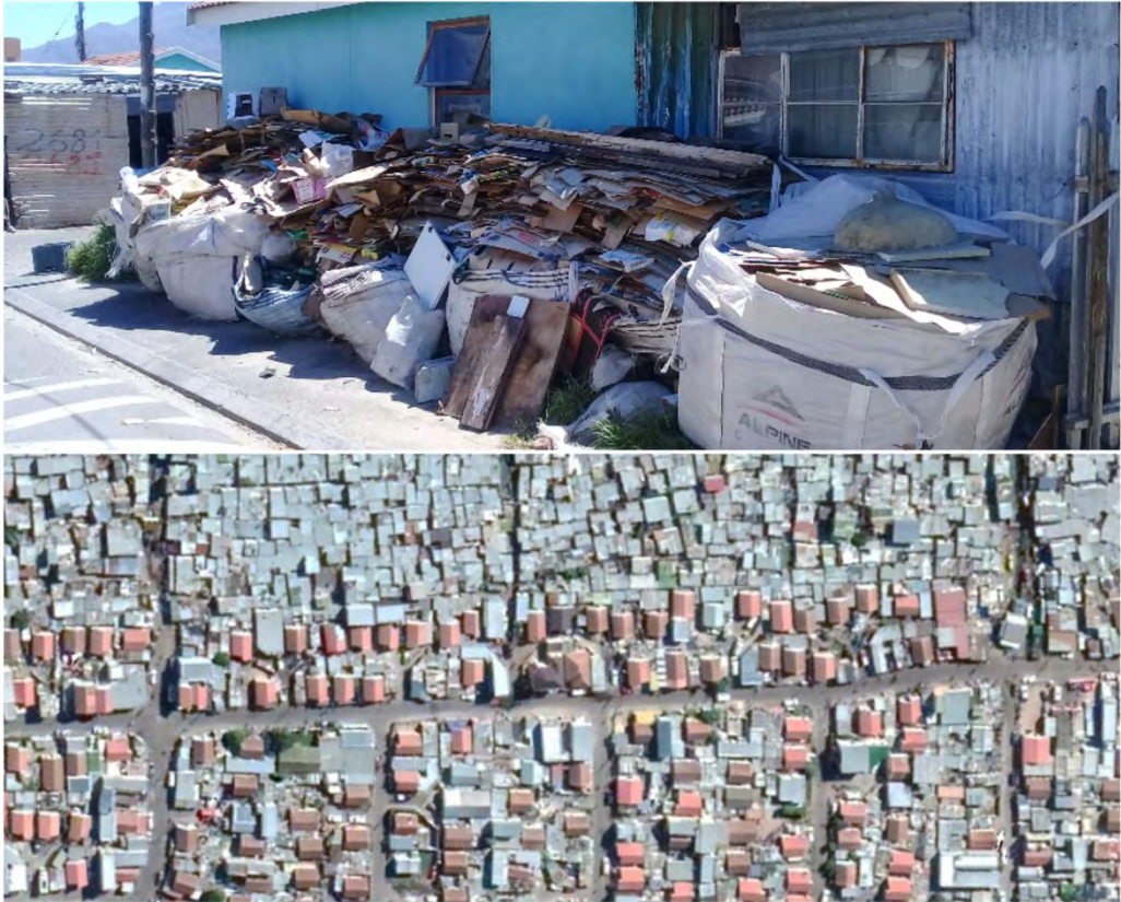
Figure 7-1: Images from Masiphumelele, Cape Town: (Top) Backyard dwelling adjacent to a formal dwelling, also depicting a high fuel load. (Bottom) Aerial view showing formal dwellings, many of which have backyard dwellings, along with a dense informal settlement (upper side of image). 78
